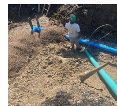
Underground line replacement
