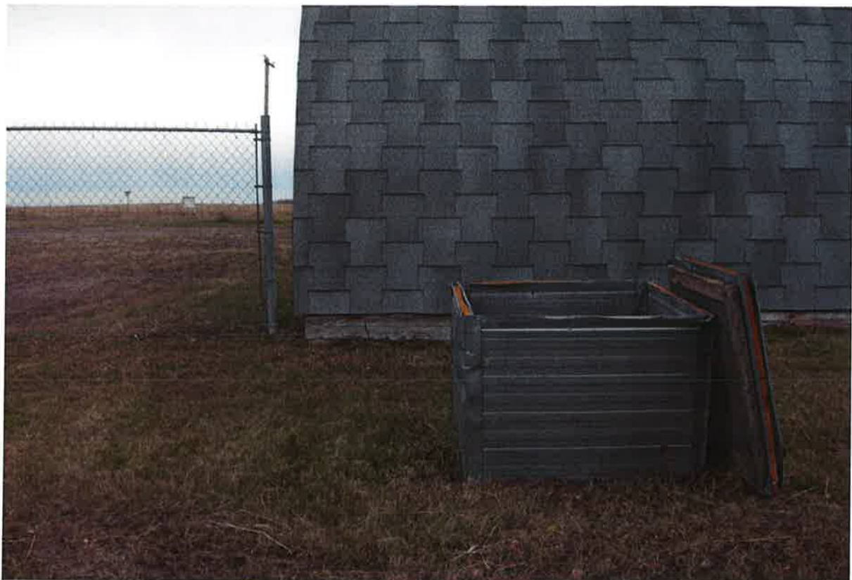
Looking north at the exterior of the septic sump (within the chain-link compound).
