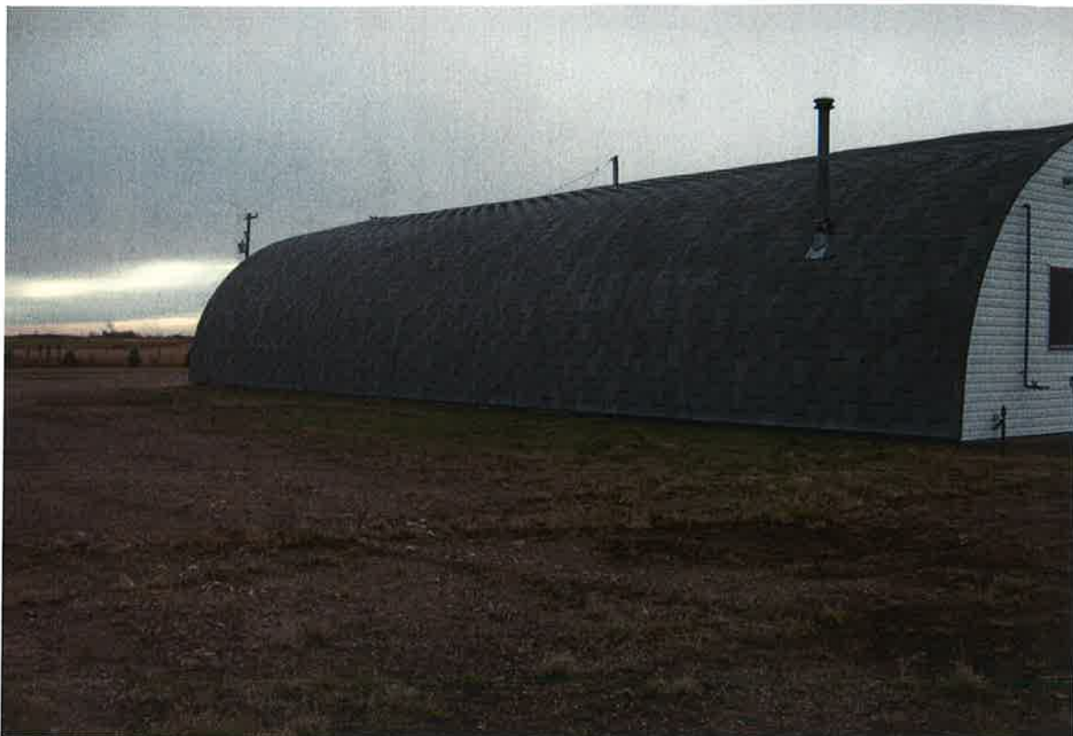
Looking at the north-facing side of the building.
