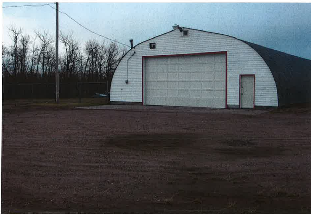
Looking at the east-facing side of the building.
