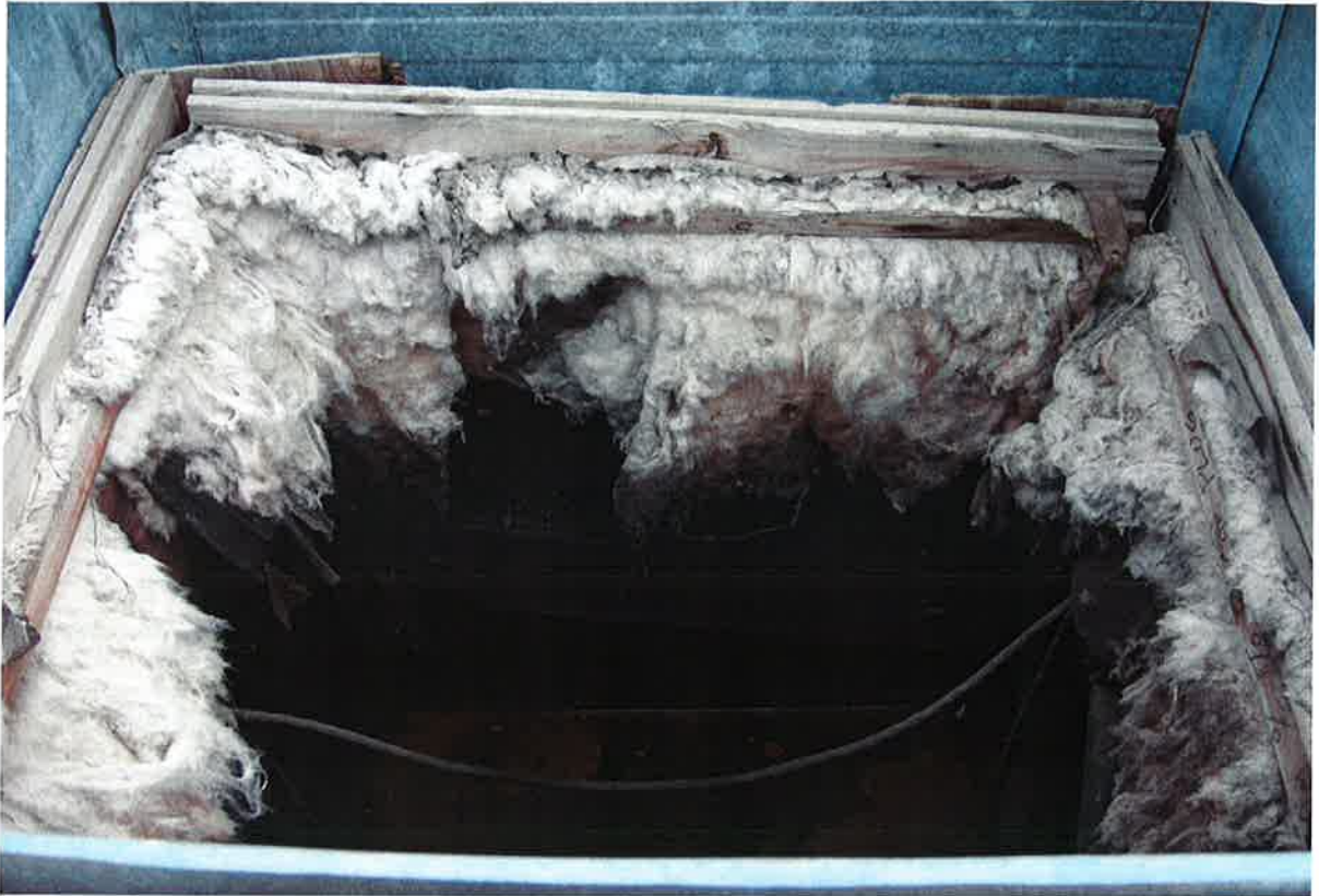
Looking at the interior of the septic sump (wood casing).
