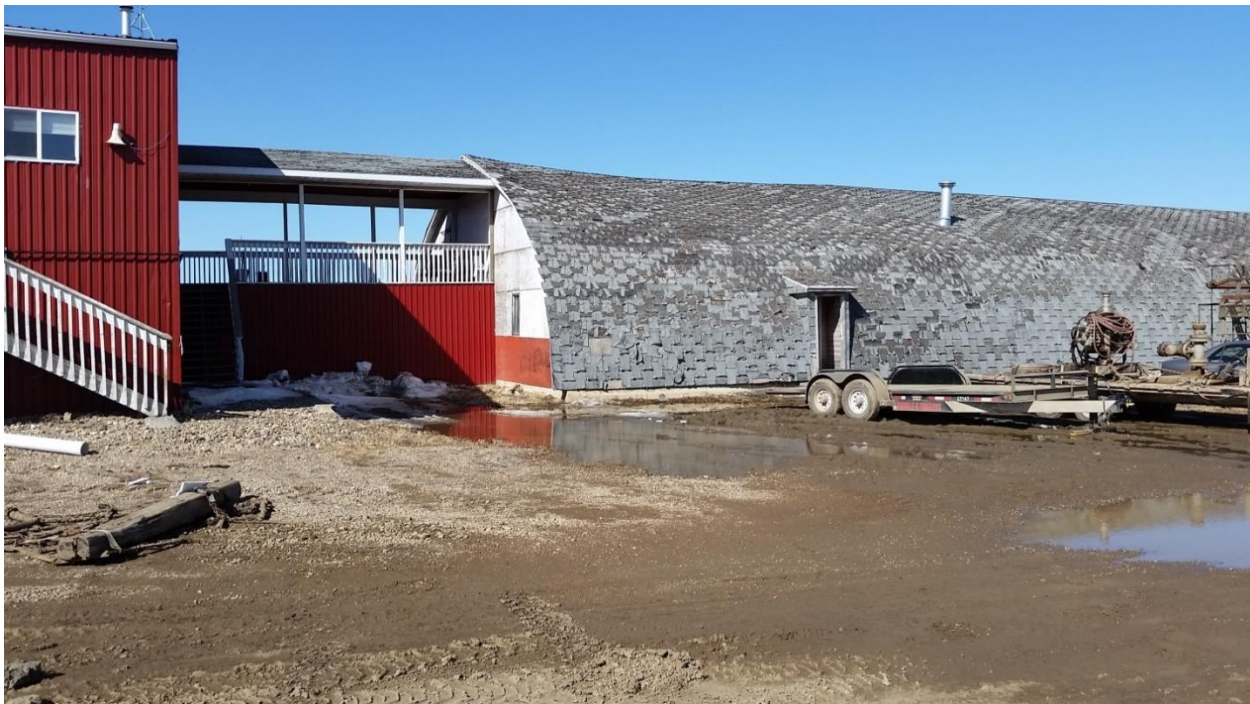
Photo 4: Site Photo Quonset (to be demolished)
