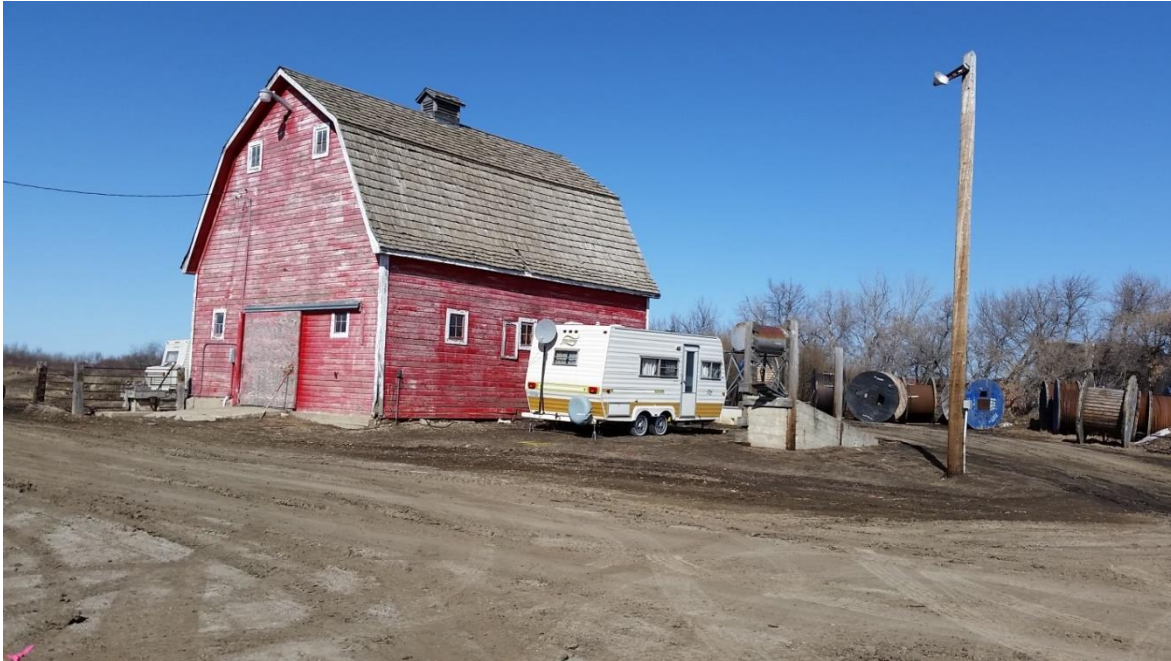
Photo 5: Site Photo Barn (to be demolished)
