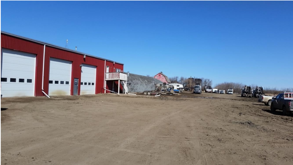
Photo 3: Site Photo Building 'G'
