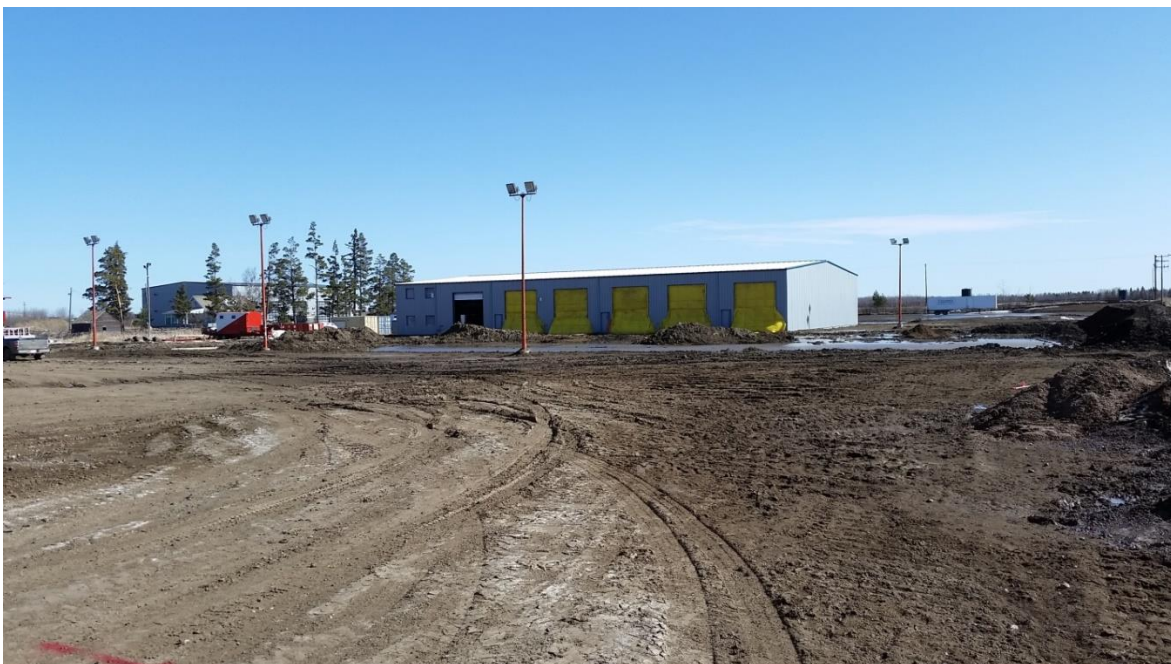
Photo 2: Site Photo Building 'C'
